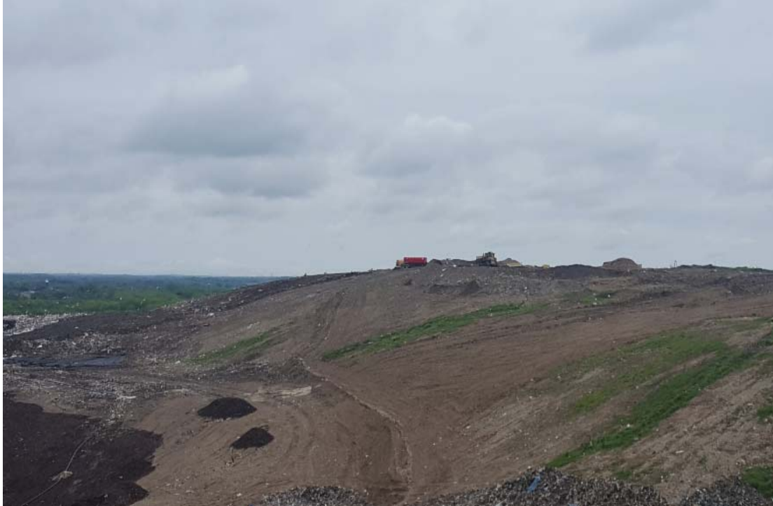
Top of Phase 6 & 7, select waste filling in settled areas
