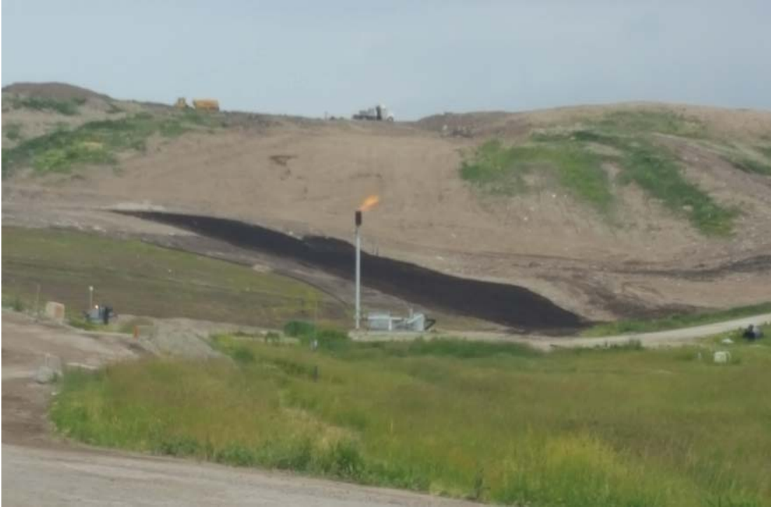
Flare at Phase 8 toe of slope.
