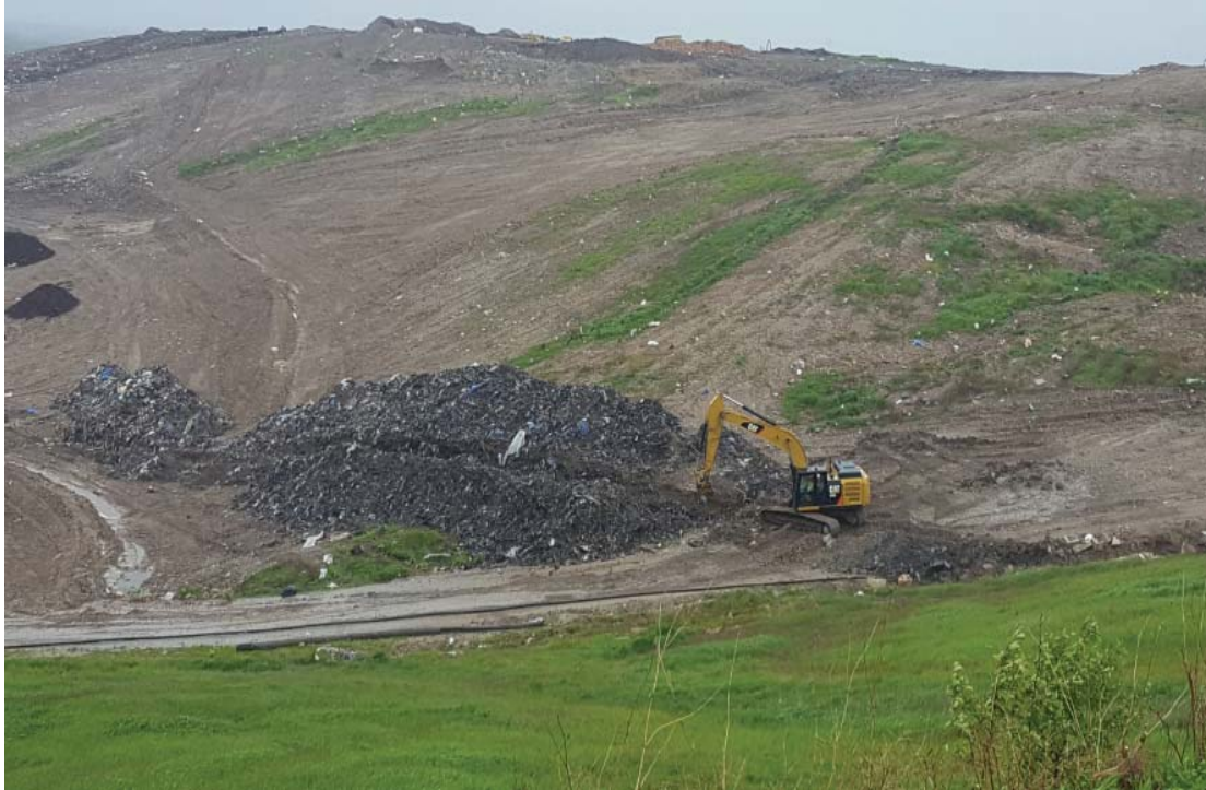
Trenching to repair seep with pipe system
