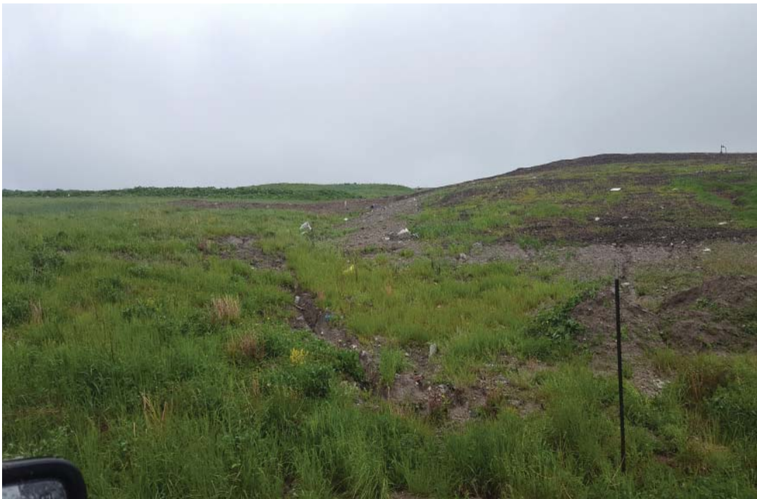
Junction the East slope of Phase 7 between intermediate cover and final cover
