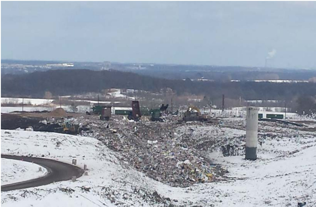
Working face at junction of Phase 8 & 9, on slope bringing Phase 8 up to grade with Phase 9
