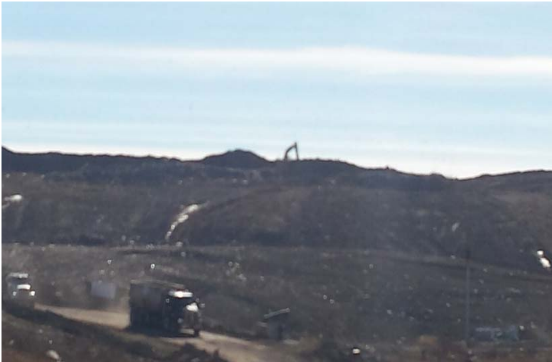
Phase 6 viewed from the North, Excavator harvesting cured bio soil for daily cover
