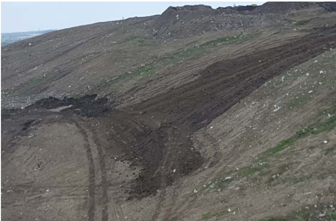
Development of diversion berms on Phases 6 & 7
