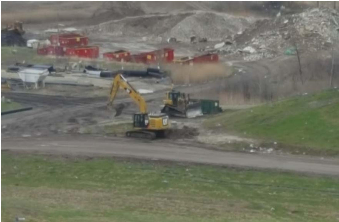
Ditch cleaning at Southwest corner of Phase 9
