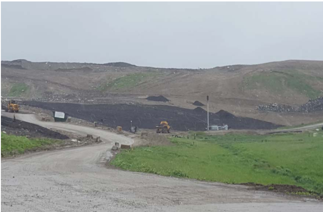
Compost placed on slope for seeding
