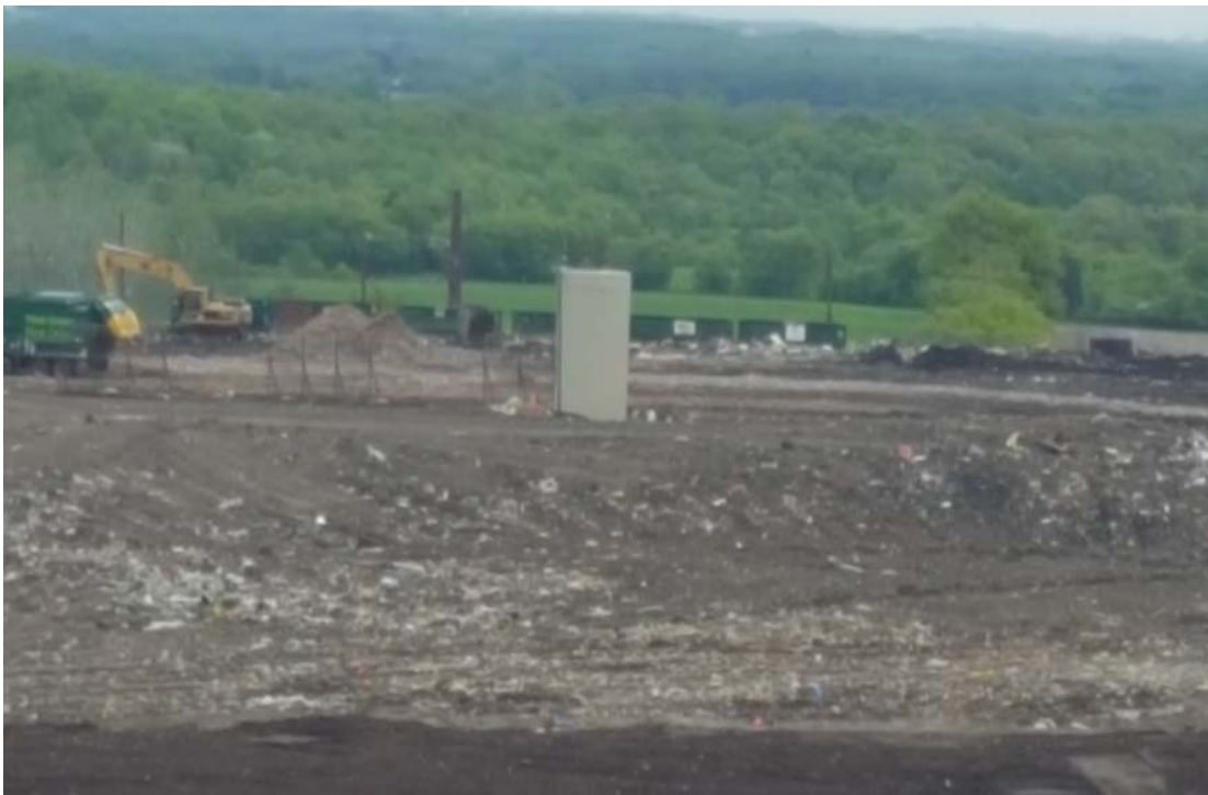
Manhole in Phase 8, waste level nearly to top
