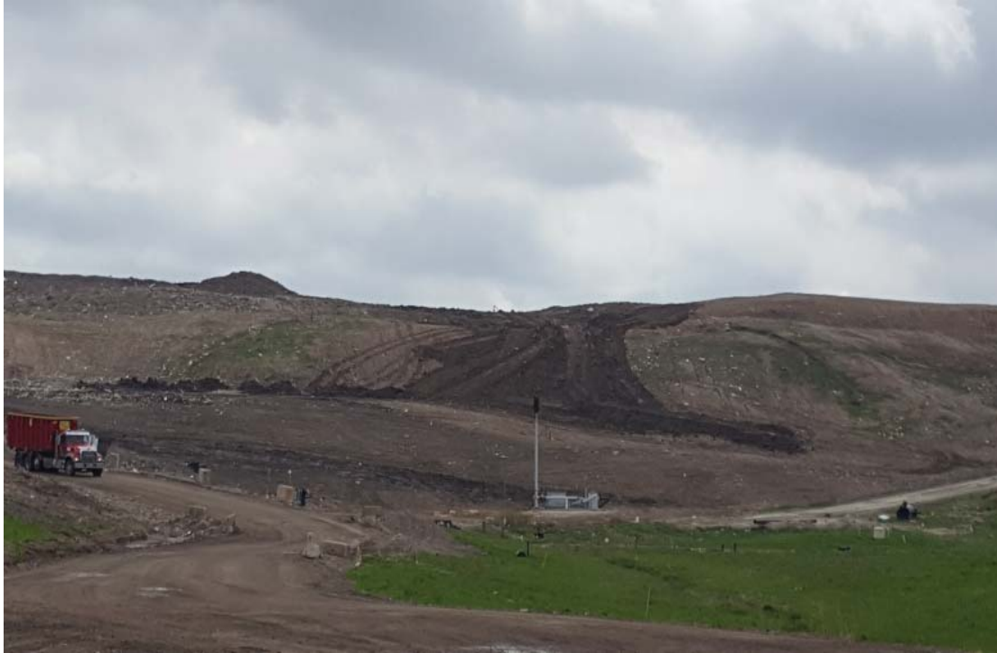
North slope of Phase 6, extra soil being harvested and used to make diversion berms
