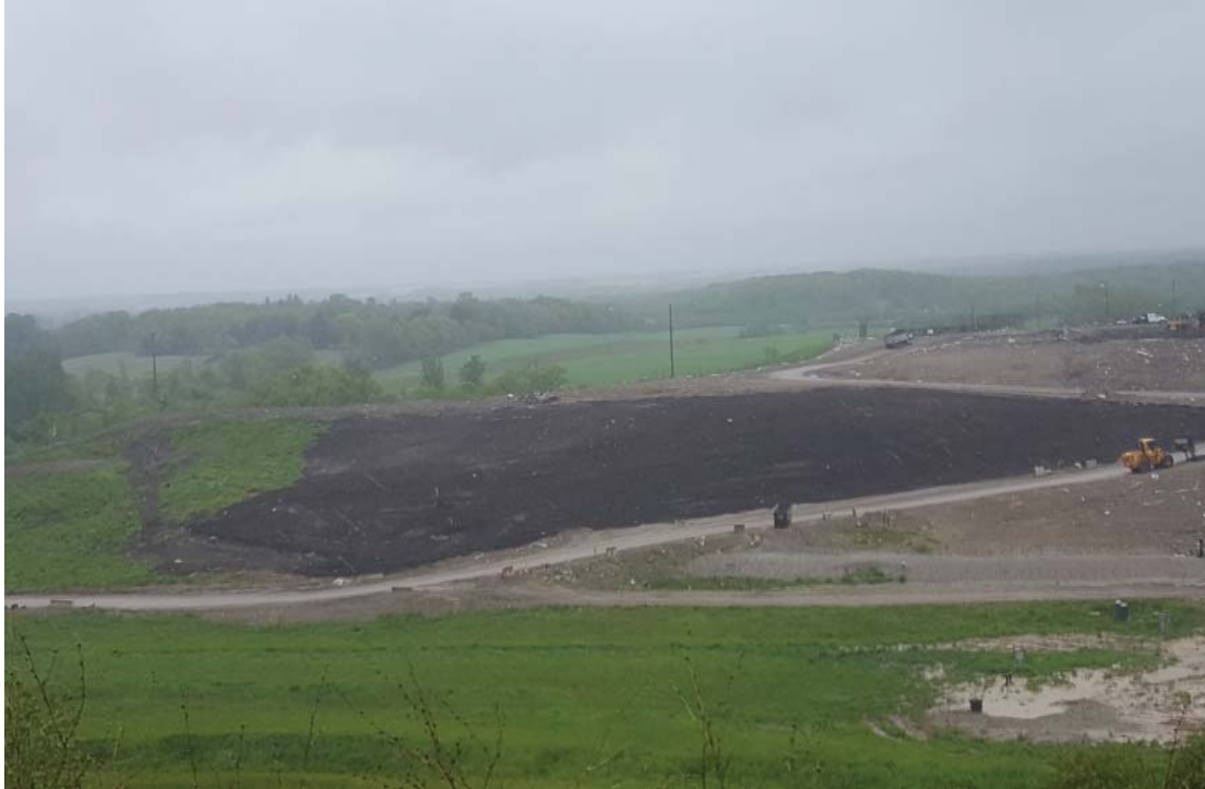
Compost placed on slope for seeding
