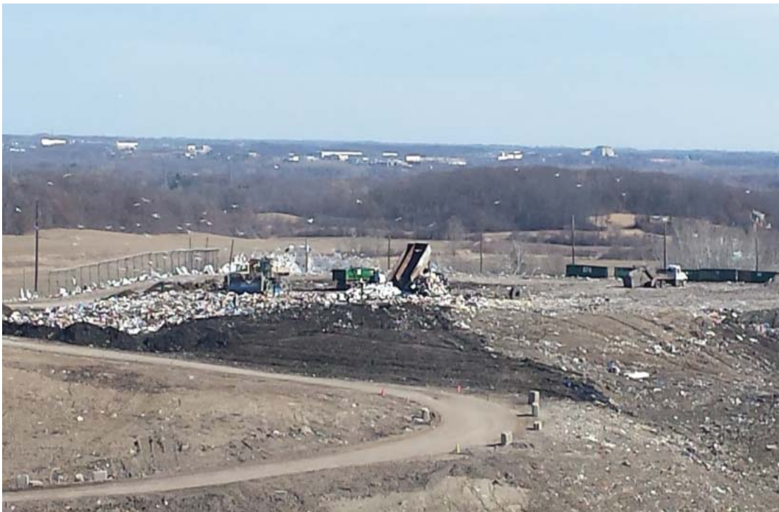
Working face in middle of Phase 8 at top of slope, soils recovered from bio pile for cover
