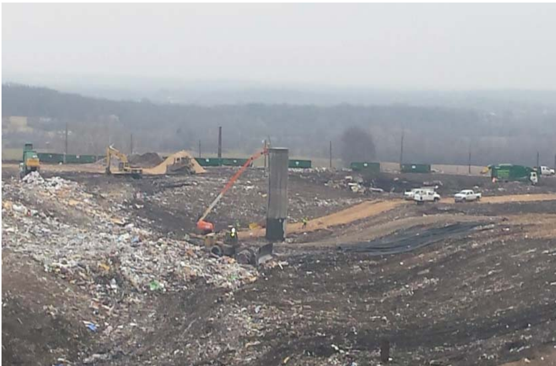
Manhole being finalized in Phase 8
