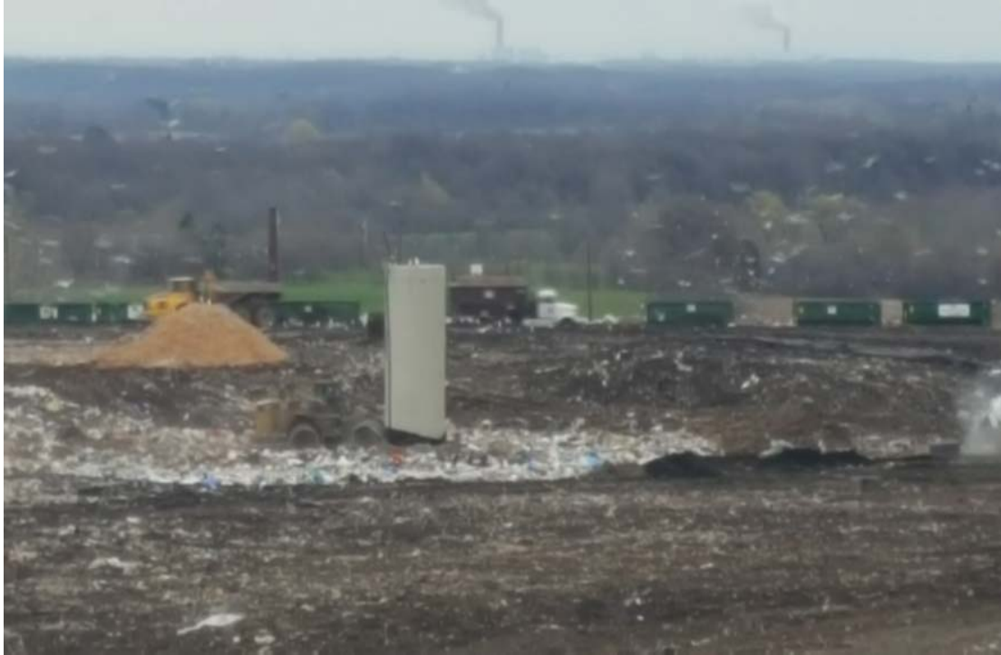
Waste about manhole brought up to grade with surrounding lifts
