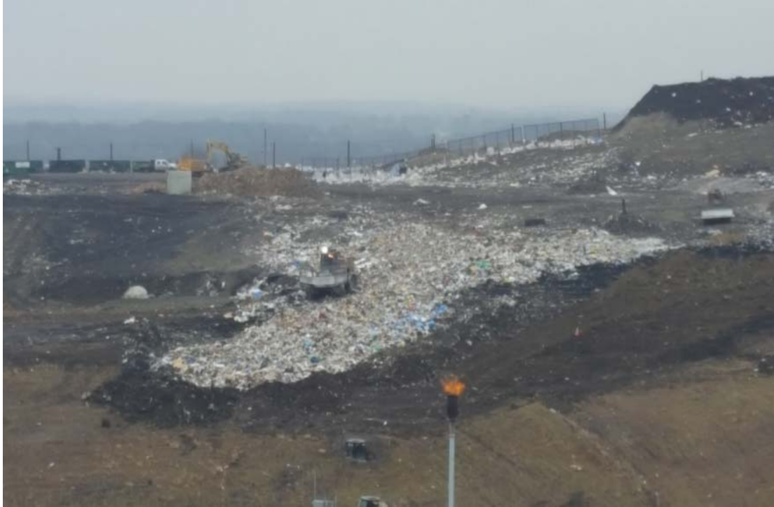
Working face, bring lift elevations up between Phases 8 and 7
