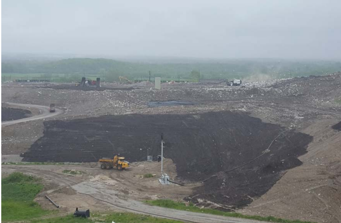
Compost placed on slope for seeding
