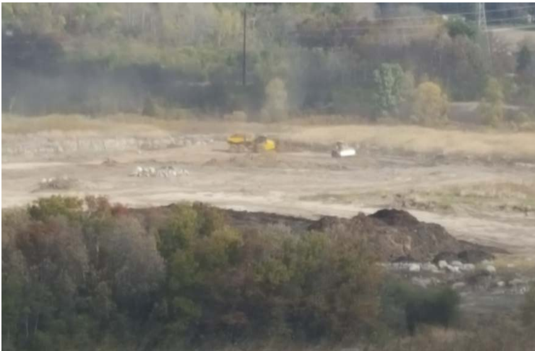
Borrow area in Northeast section of Landfill. Stockpiling top soil closer to camera, clay being tipped in far North West corner
