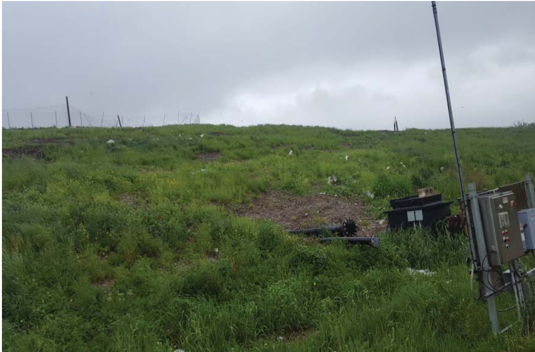
East slope of Phase 8 & 9, erosion will require repairs in dryer weather
