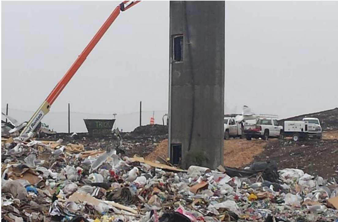
Manhole, final connection and closing of openings ongoing today
